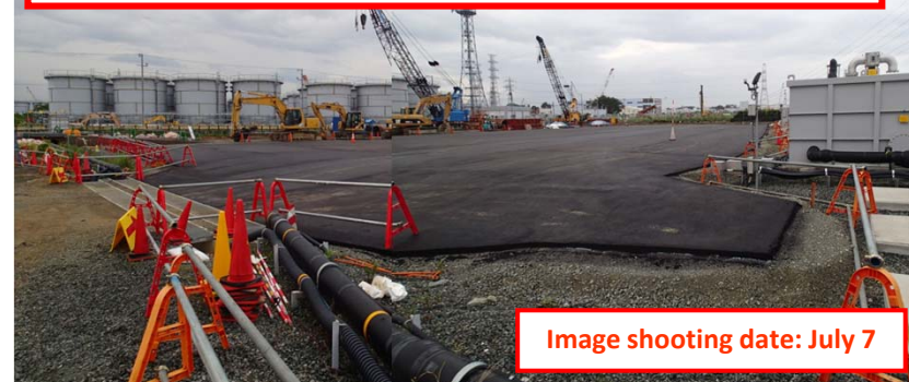
After asphalt pavement works completion (partial)
