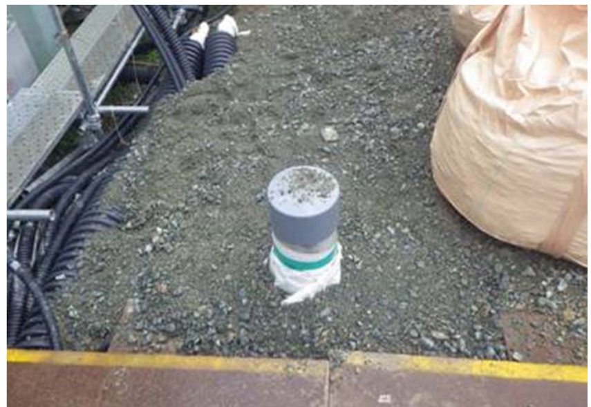
Pit for new subdrain N12
