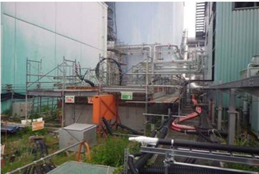
Foundation work for relay tank #3
