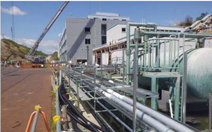
Setting up transfer pipe (north side of Unit 1)
