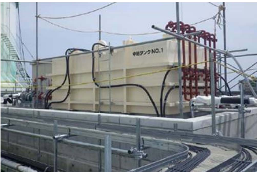
Setting up relay tank #1
