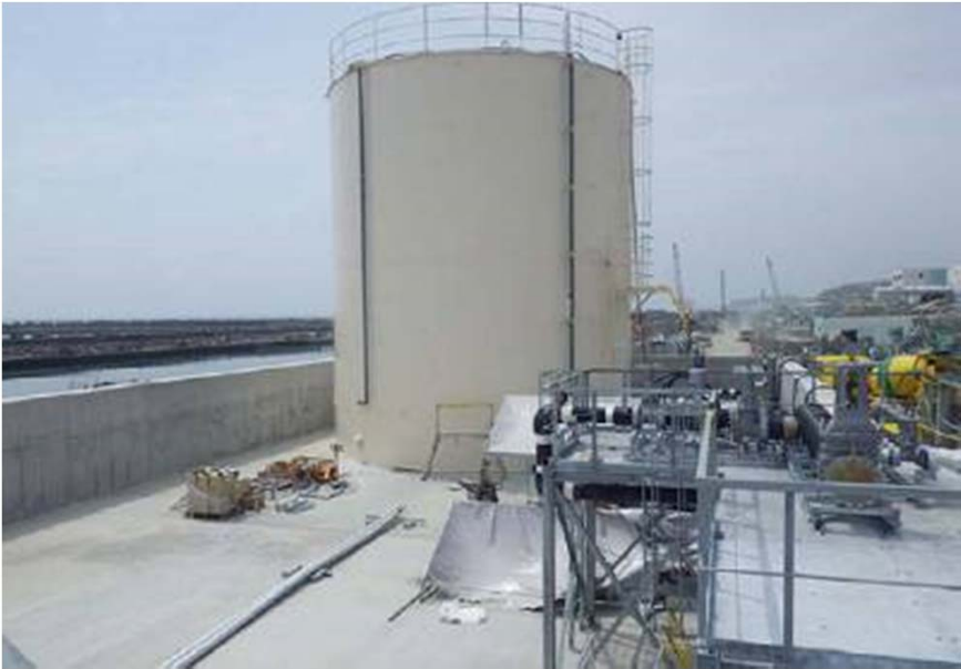
Setting up catchment tank
