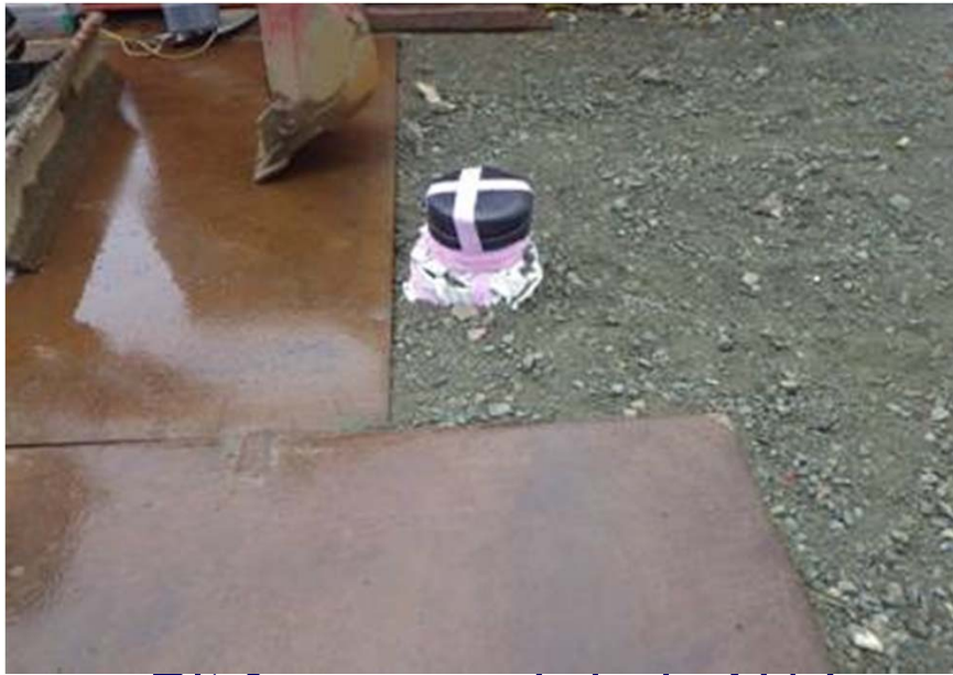
Pit for new subdrain N14
