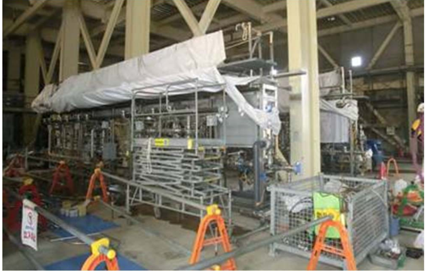
Setting up pre-processing skid
