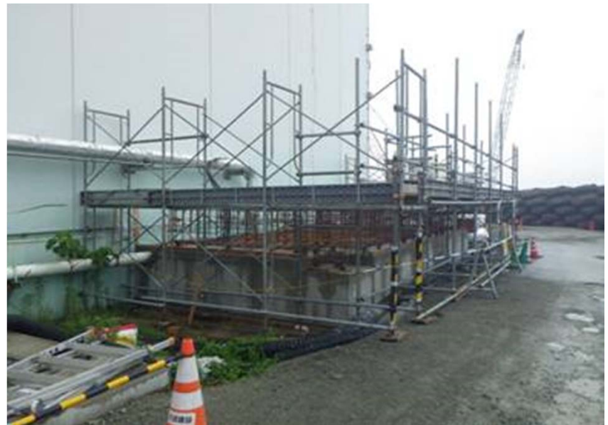
Foundation work for relay tank #5
