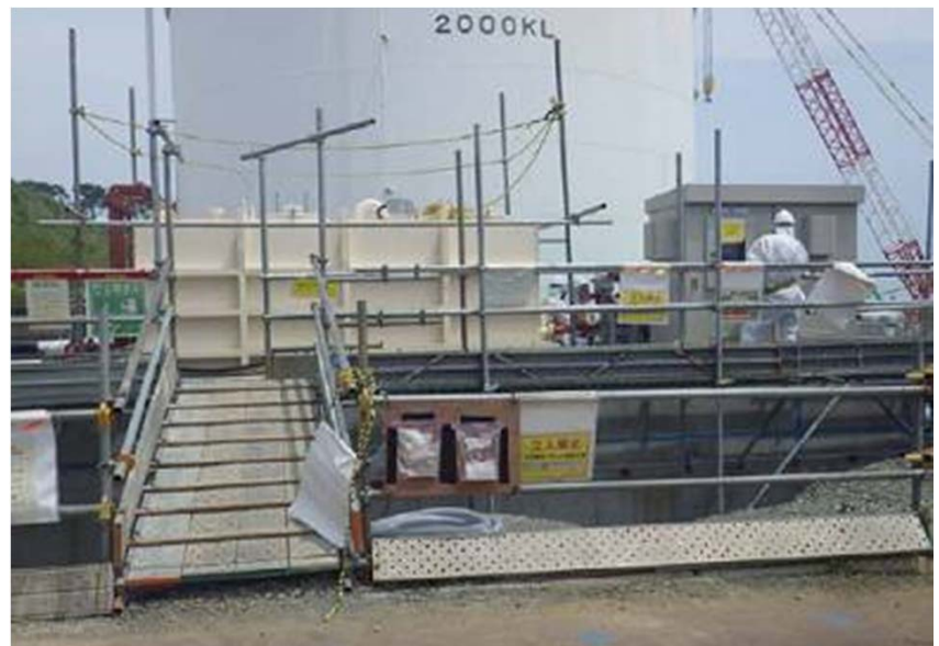
Setting up relay tank #2
