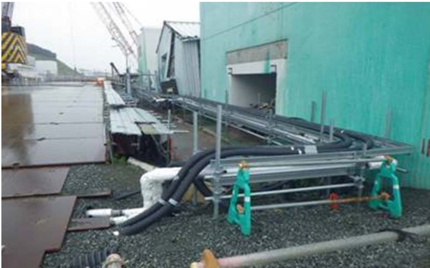
Setting up transfer pipe (east side of Unit 1)
