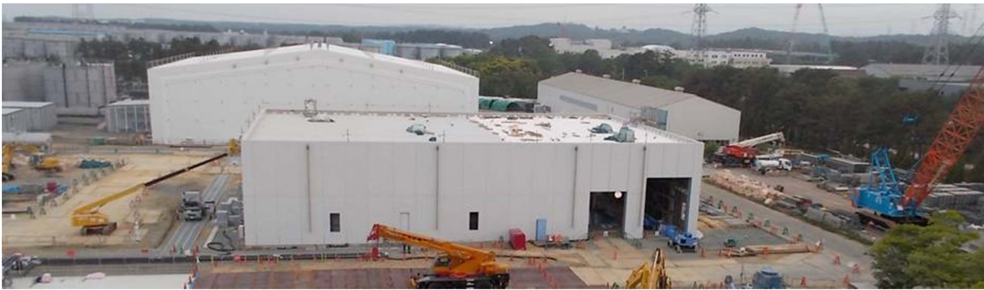
Construction site panorama (north side)
