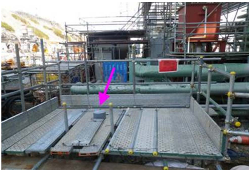
Pit for new subdrain N9
