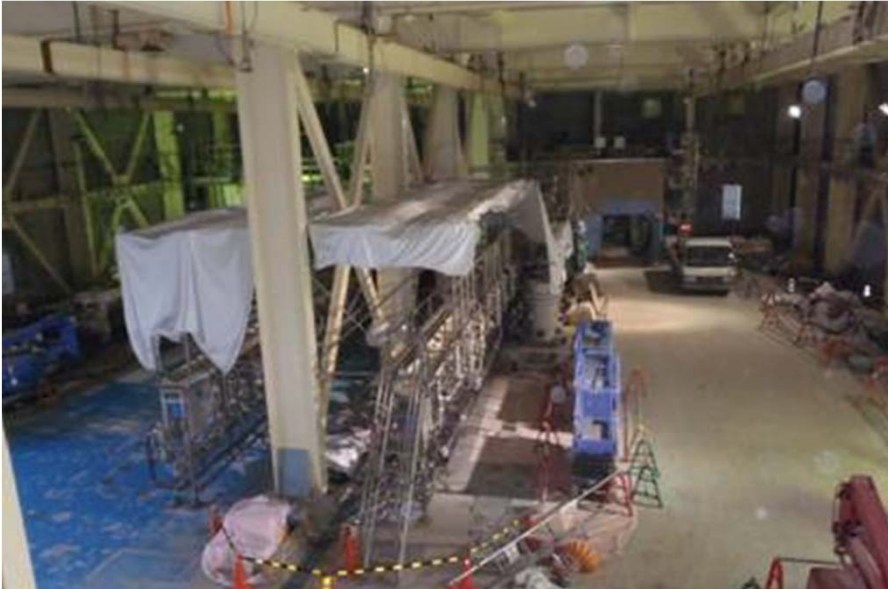
interior of the building
