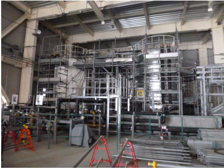
Setting up supply tank for treatment system
