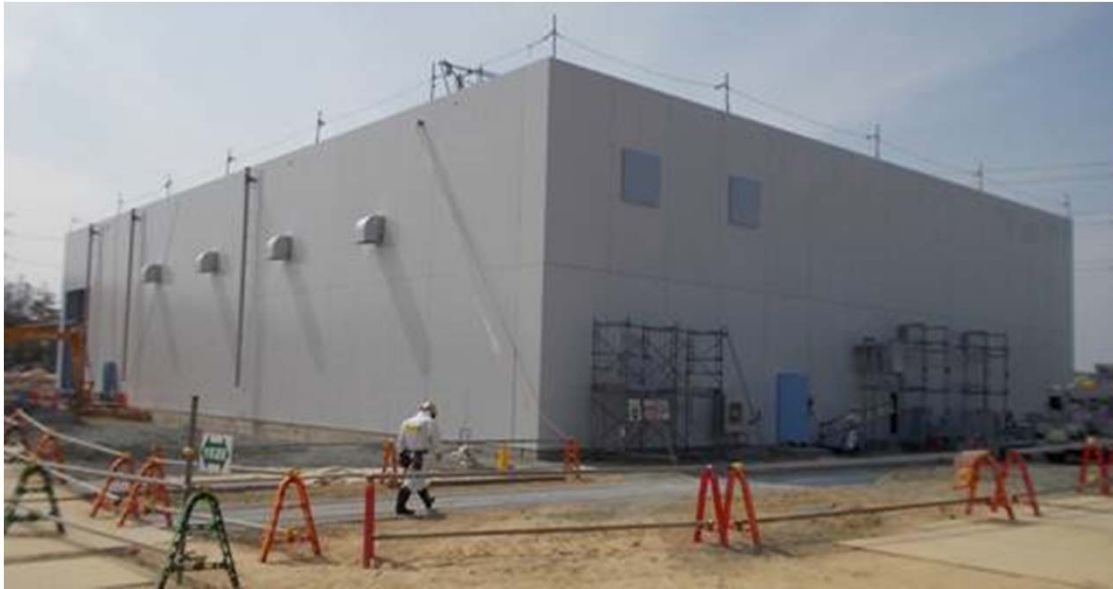
exterior of the building (southeast side)
