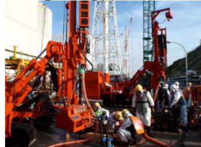
Installing freezing pipes
