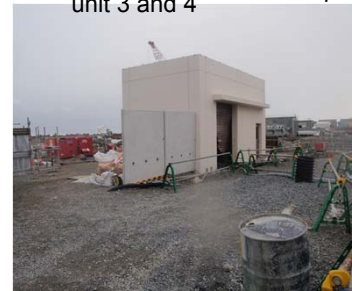
Sea-side between unit 3 and 4 before operation
