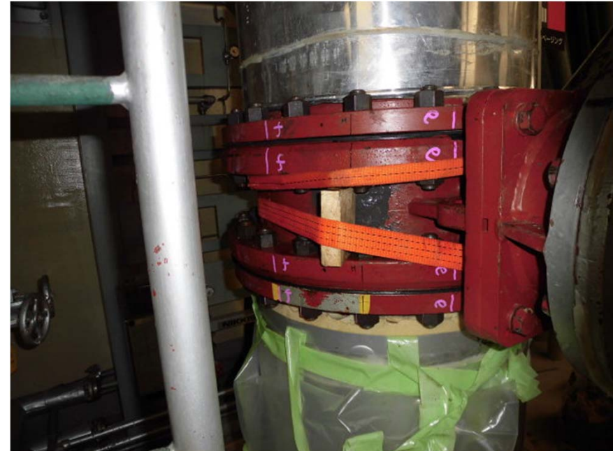
[2] Provisional repair with hardening agent
