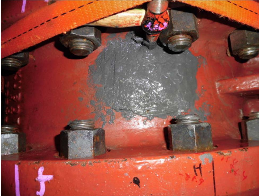
[1] Provisional repair with hardening agent
