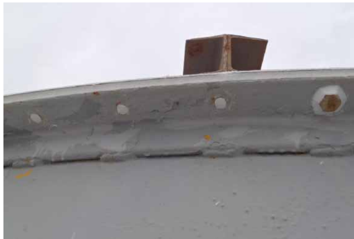
Caulking treatment for the top plate at B south tank area
