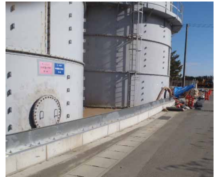
Dike raised upward at B south tank area
