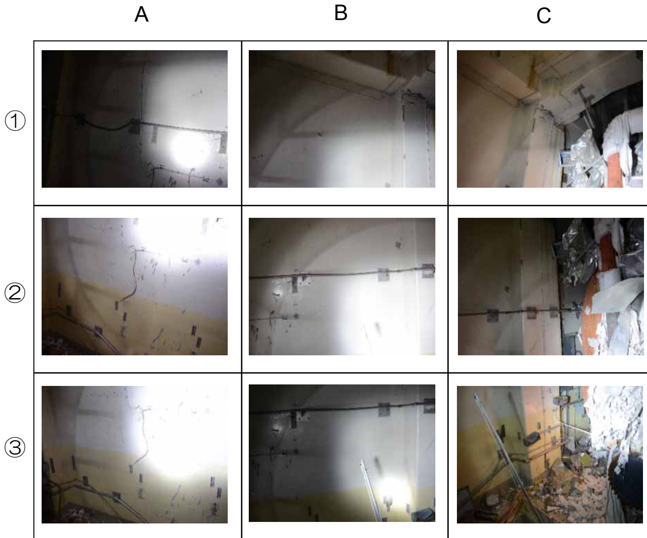
[4th floor equipment hatch walls in the west]
