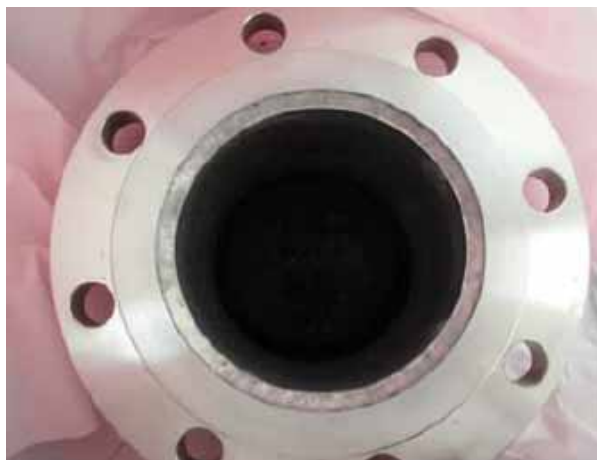
⑨ Adsorbent tower 2C inspection hole
