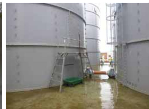
Installation of receiving pan
