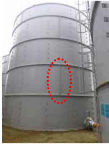
Location where the leakage was found
