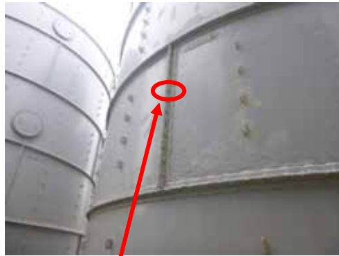
Location where the leakage was found
