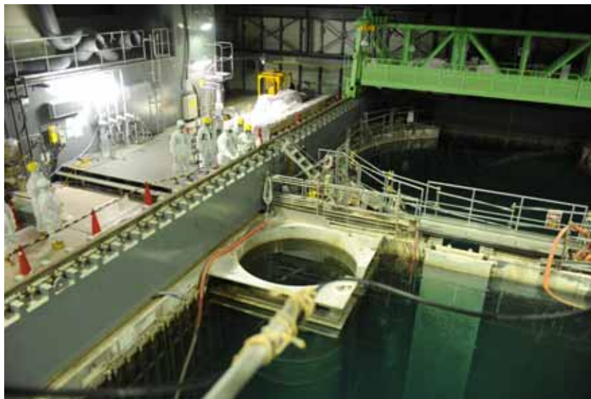
Observation of the Unit 4 spent fuel pool
