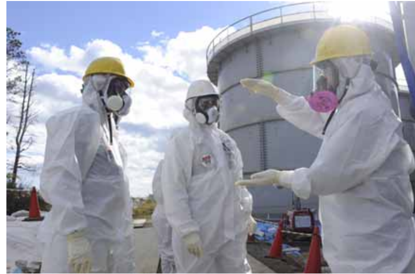
Observation of the tank area
