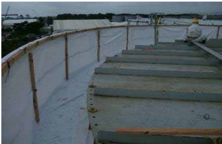
Foothold of the tank No.3
