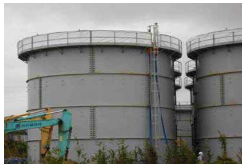
Full view of the tank No.12
