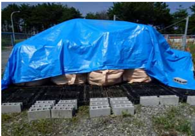
Flexible container bags covered with protection sheet
