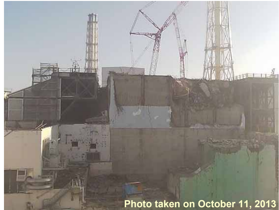
After large debris removal
