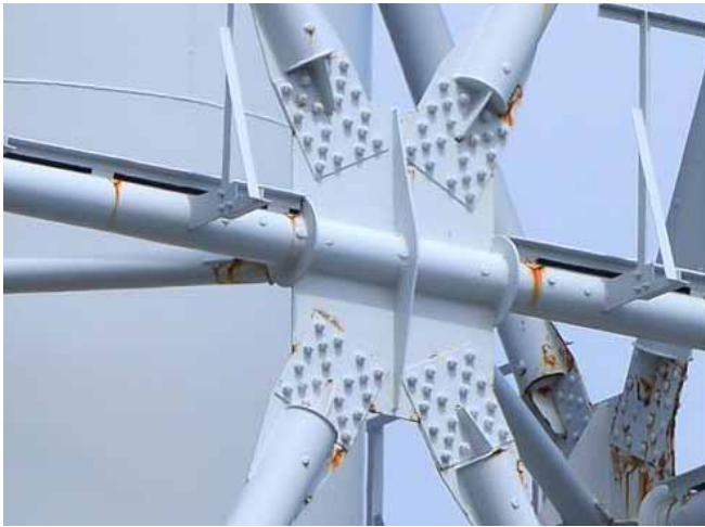
① South side (around 100 m above ground) A joint section
