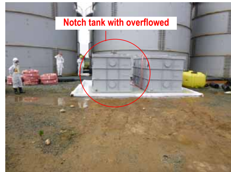
Photo taken by TEPCO on October 1, 2013
