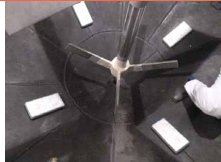
Batch treatment tank 1C (after rubber lining was provided)
