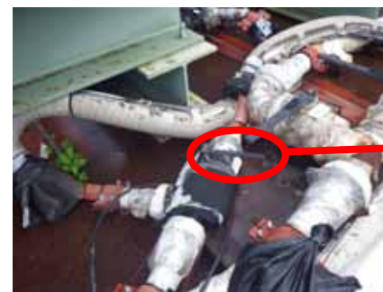
Main valve of treated water storage tanks
