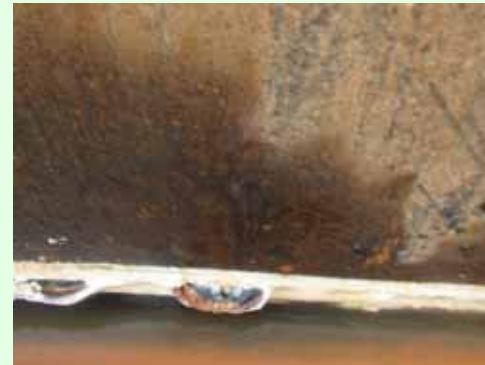
No.10 Sealed part (Photo taken on Sep. 15, 2013)
