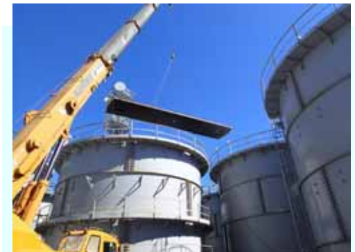
No.5 Top plate removal (Photo taken on Sep. 17, 2013)
