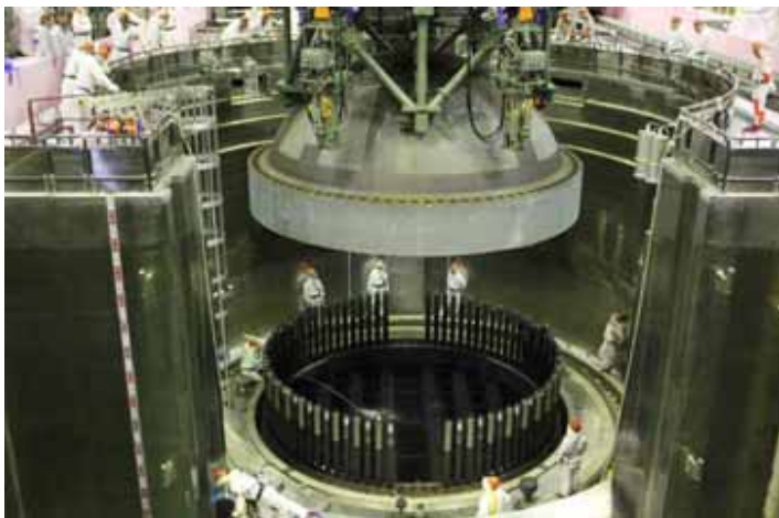
<Reference> Work progress on lid removal from the reactor pressure vessel (Unit 4 at Fukushima Daiichi NPS)
