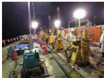
<Foundation improvement work>
