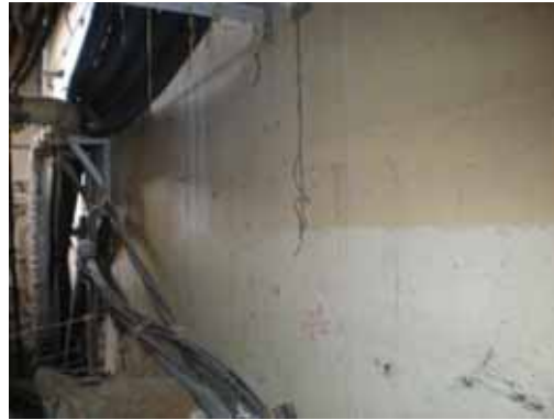
⑥ SFP side wall (East side)
