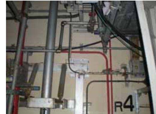
④ West wall (Inner surface)
