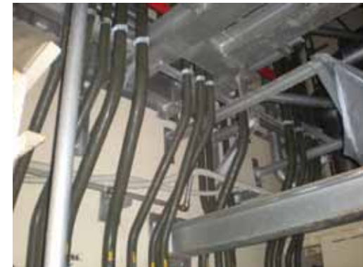
② South wall
