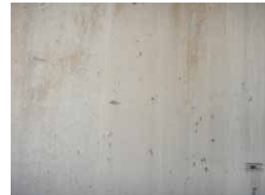
⑨ SFP side wall (West side)
