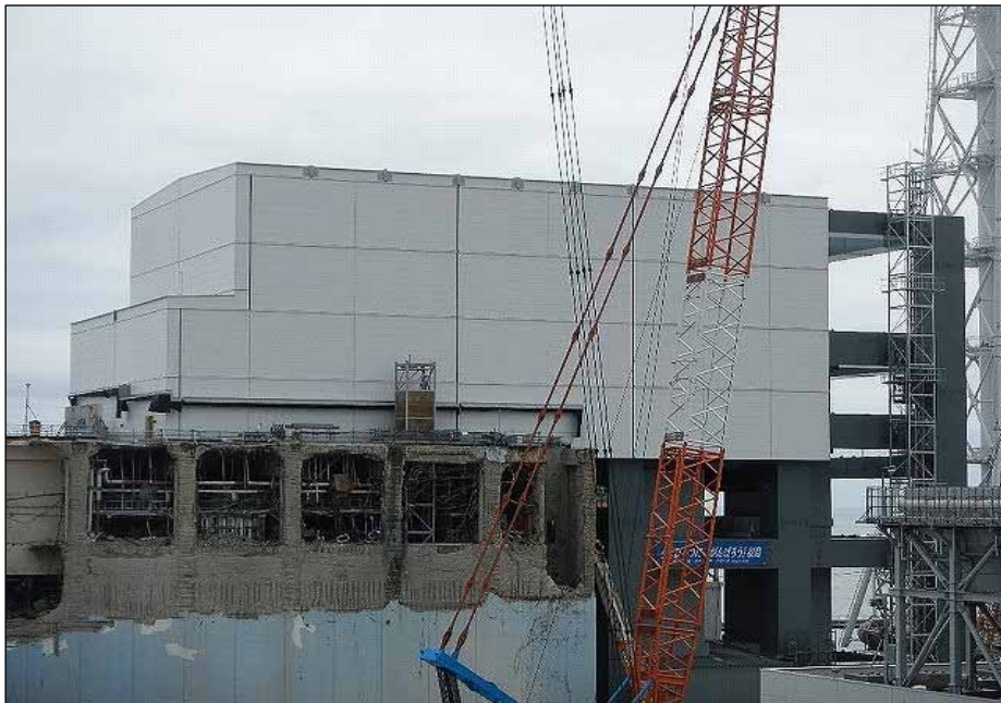
Completion of outer wall and roof panel installation (July 20)
