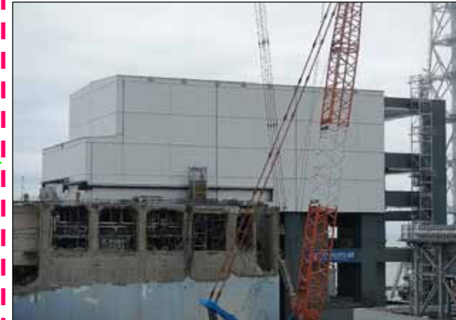
(5) Completion of outer wall and roof panel installation (July 20, 2013)
