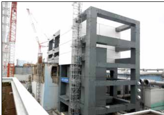
(4) Completion of the steel frame construction (May 29, 2013)
