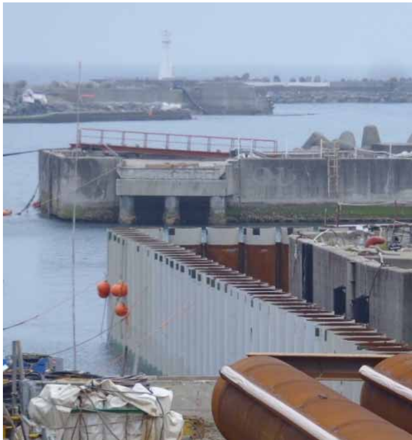
Condition at the north side of Unit 1-4 water intake channel
