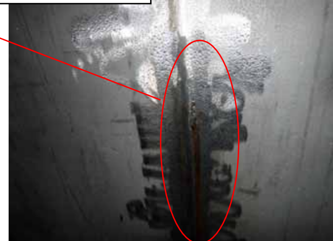
(1) Condition at the bottom part of the tank (enlarged image)
