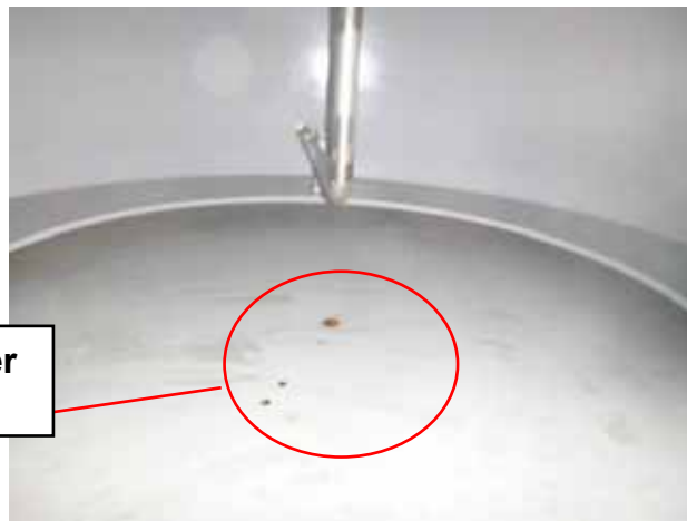
(2) Condition of the leaked water receiving pan
