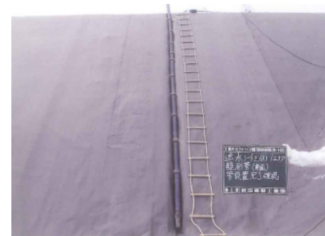
Conceptual drawing of installation of detection hole/ deformation and damage, photo of installation
