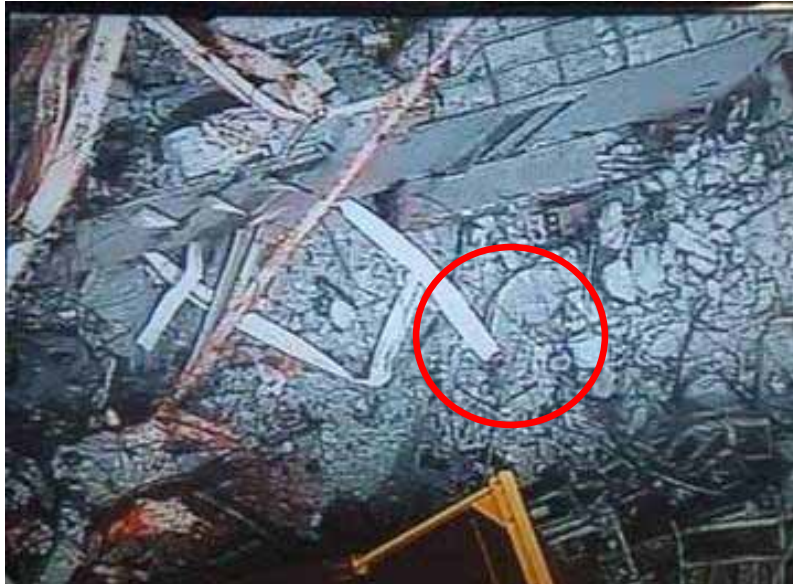
1. Before work (April 17, 2013)
