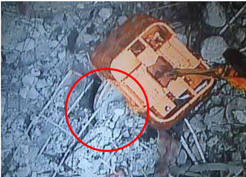
2. During work (April 18, 2013)
