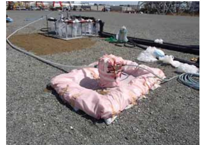
Installation of the pump at underground reservoir No. iii (photo taken on April 13)
