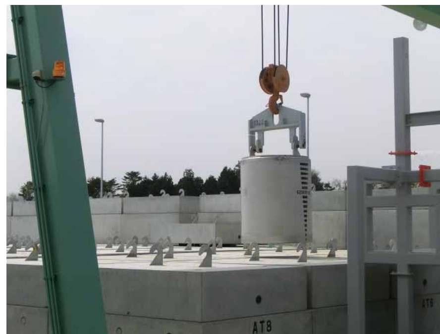
Temporary storage facility area
