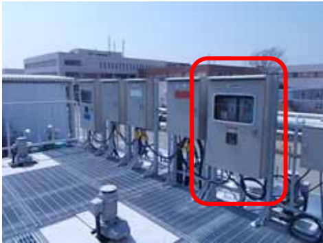
The control panel of the Standby Liquid Control System Tank Heater A (Upper part of the Standby Liquid Control System Tank A)
