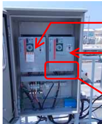
The control panel of the Standby Liquid Control System Tank Heater A (Upper part of the Standby Liquid Control System Tank A)
