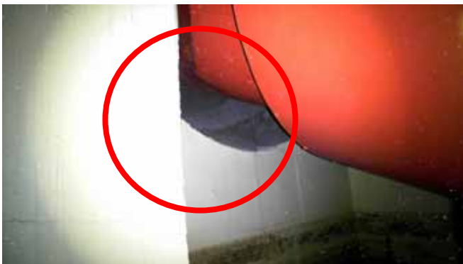
Edge of the vent pipe sleeve
