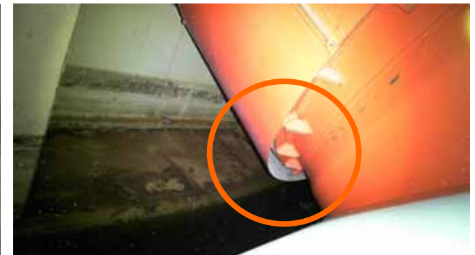
Lower part of the vent pipe bellows cover
