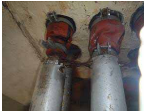
Pipe penetration area before water stop work (duct side)
