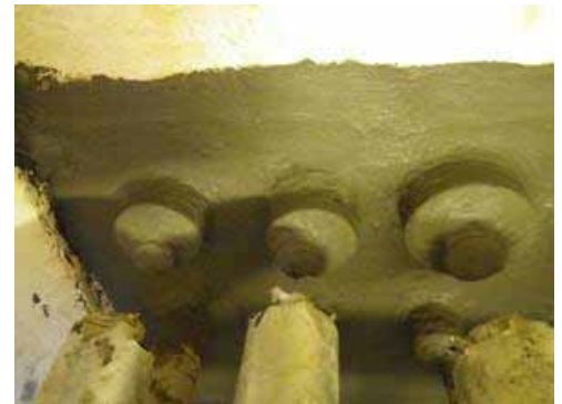
Pipe penetration area after water stop work implementation (duct side)
