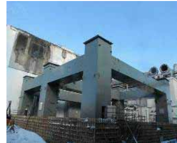
The first layer of steel framing completed (January 14)
