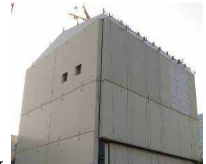
Installation of Unit 1 reactor building cover
