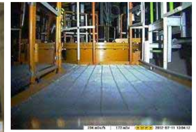
Investigation of the torus room by using robots (July 11, 2012)
