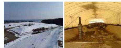
Condition of 1st facility (Photo taken on January 16)
