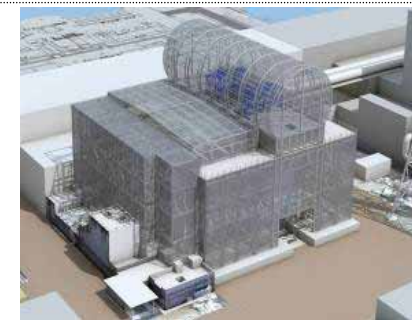
Simulated image of the cover to be installed for fuel removal
