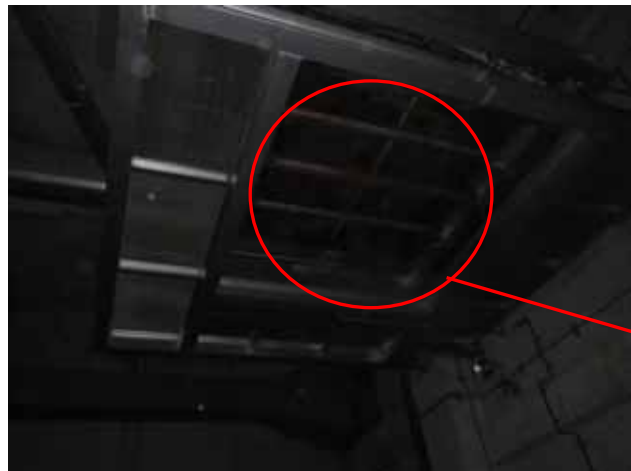
Ceiling on the second floor (Photo taken on February 25 by TEPCO)
