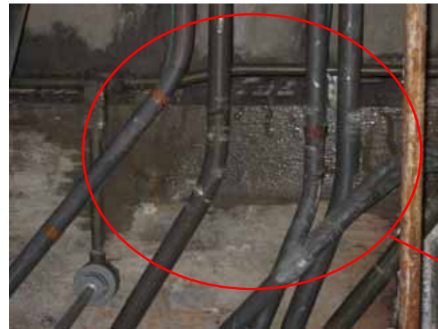
Ceiling on the first floor (Photo taken on February 23 by TEPCO)
