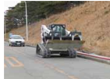
Heavy machinery heading to the site
