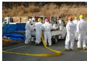
Starting water injection (in front of the Water Treatment Building)
