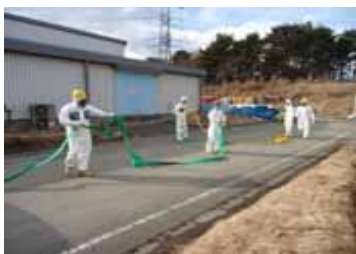
Preparation for injection (in front of the Water Treatment Building)
