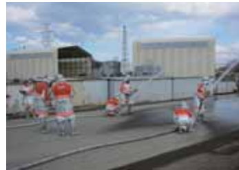
Fire fighting at the site (in front of the large equipment inspection building)
