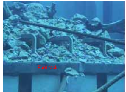
Photo 3: Sediments on the fuel rack
