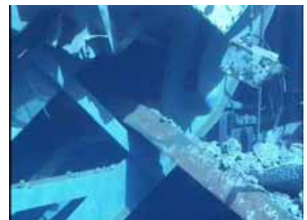
Photo 5: Bridge of the fuel handling machine
