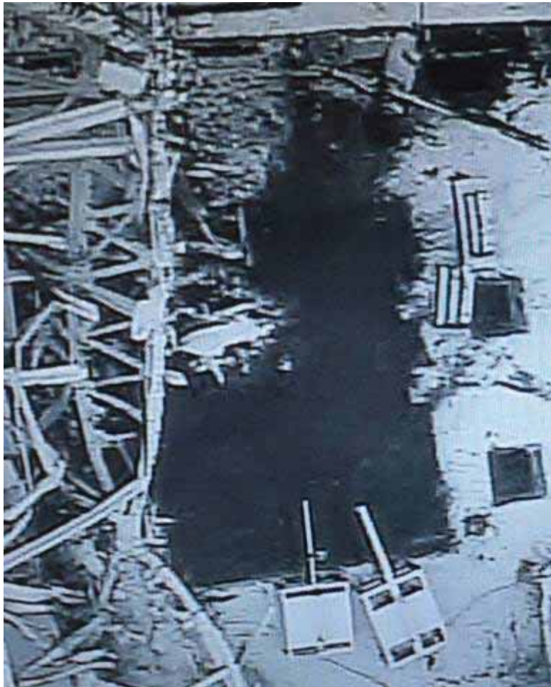
Spent fuel pool (after steel truss removal)
