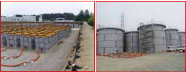
Fresh Water, RO Concentration Tanks
