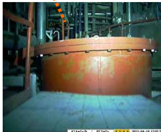
Survey inside the Unit 2's torus (April 18, 2012)
