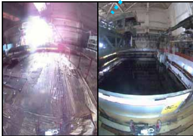
Survey on 5th floor in Unit 2 R/B (June 13, 2012)
