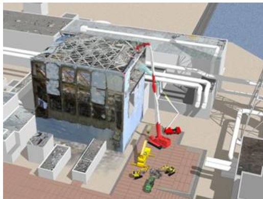
Debris removal from the upper part of reactor building
