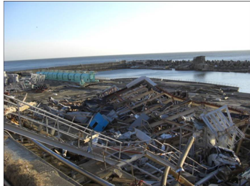
Unit 5,6 Intake Screen Area
