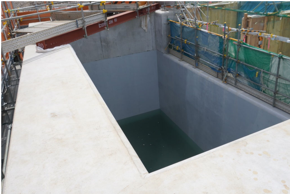
Discharge vertical shaft (down-stream storage) after it has been filled with water [photo taken on June 6, 2023]
