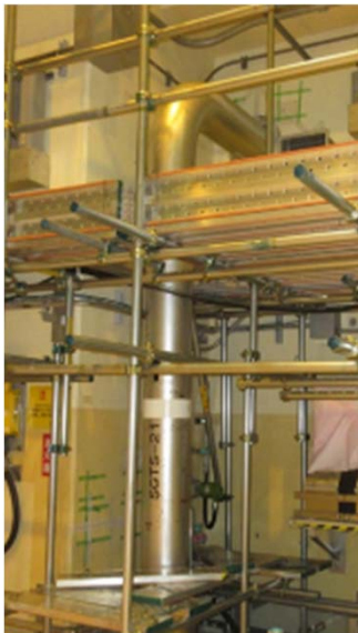
Prior to fire protection renovations
