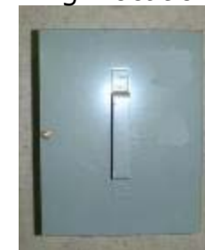
Metal box used to house electric wire conduits
