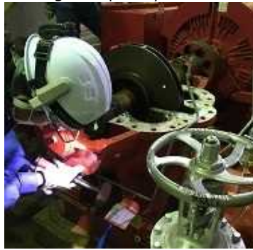
Fire pump repair training (overhaul)
