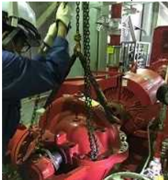
Fire pump repair training (hoisting)
