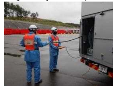
High voltage generator truck operation training (power supply team)
