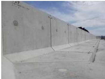
Kuril-Kamchatka Trench Tsunami Seawall
