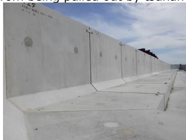
Kuril-Kamchatka Trench Tsunami Seawall
