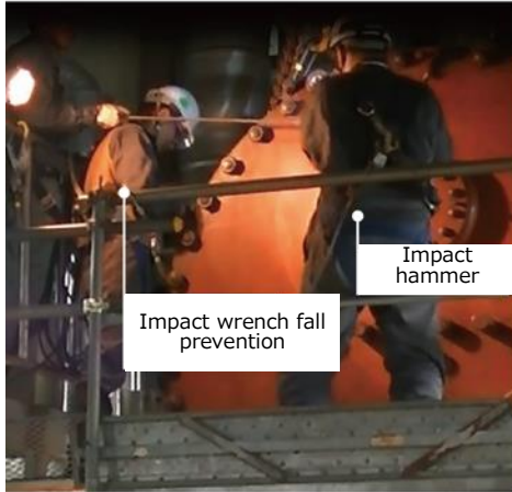
Kaizen for the removal and tightening of water chamber bolts/nuts
