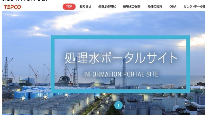
Treated water portal site
