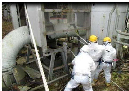
Suction pipe replacement
