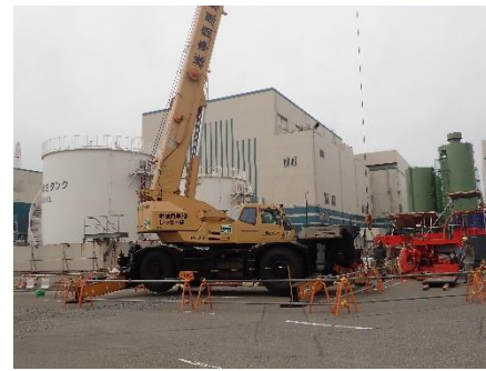
Unit 6 diesel fuel tank
