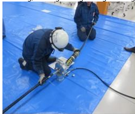
Cable terminal preparation/connection training
