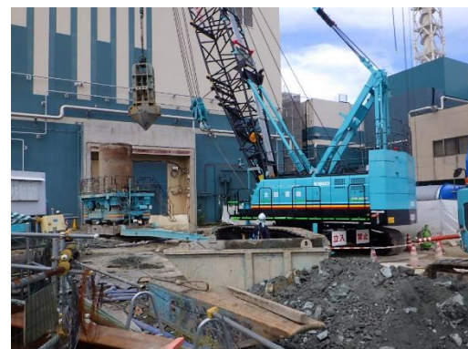
Ground improvements for the large freight entrance
