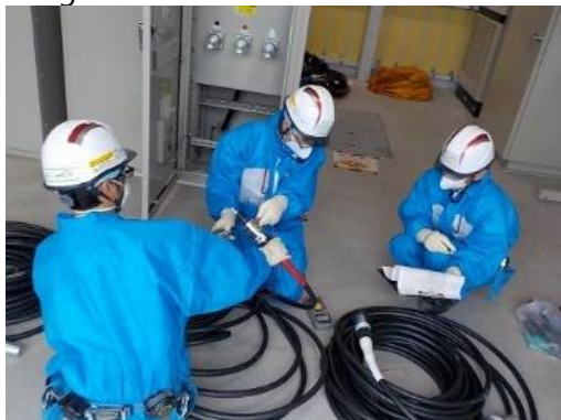
Cable conductivity check (power supply truck operation/connection training)
