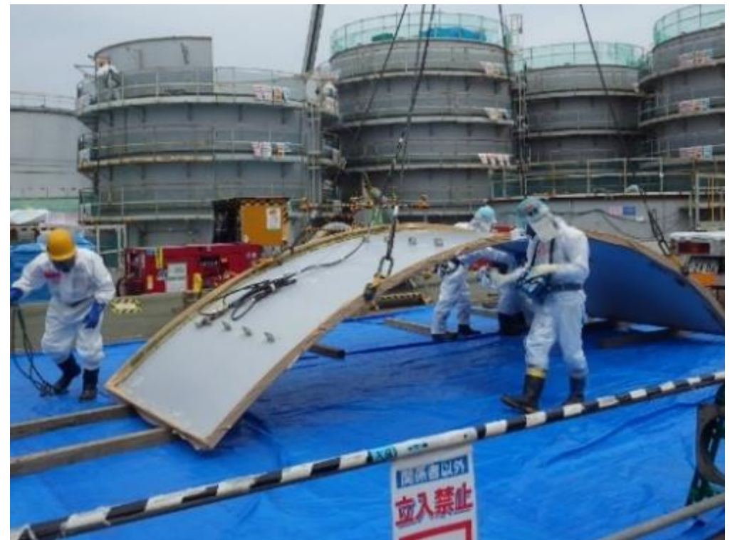
Flange tank disassembly kaizen (Fukushima Daiichi)
