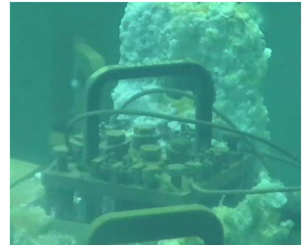
Upper section after the test (Photographed on August 18, 2026)
