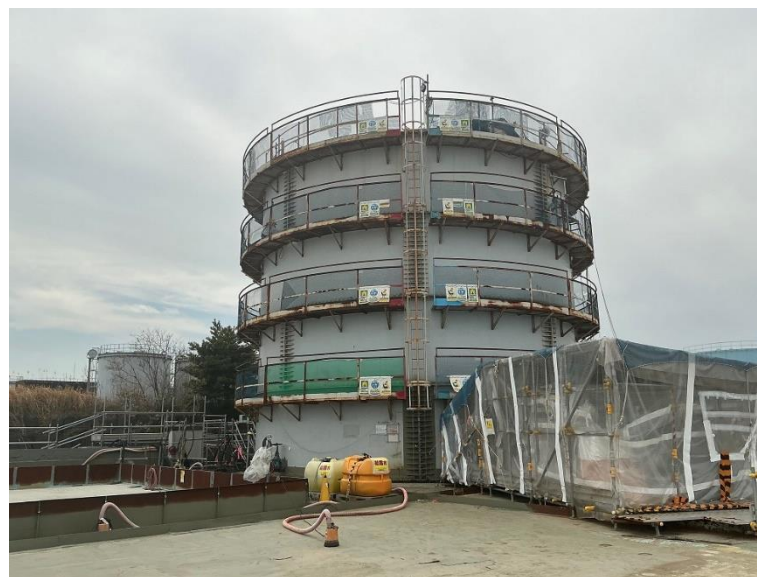
External view of D1 tank in E area (April 13, 2026)
