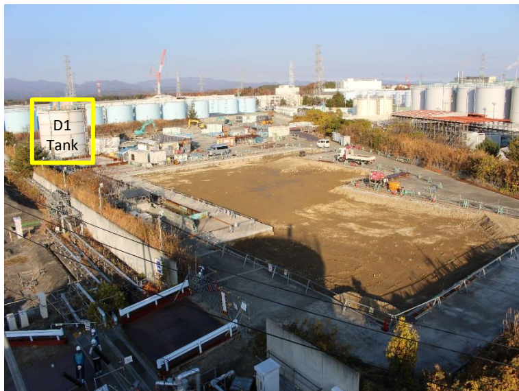
Conditions in E area (November 27,2025)
