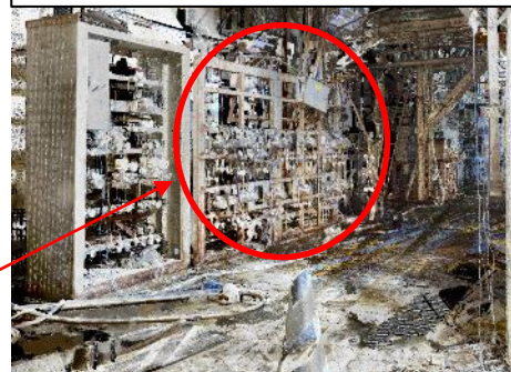
High pressure coolant injection system instrument rack (west area, 1st floor, reactor building)
