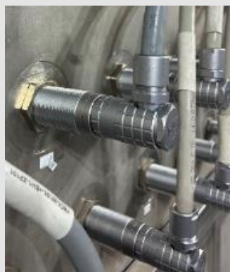
Prior to caulking
