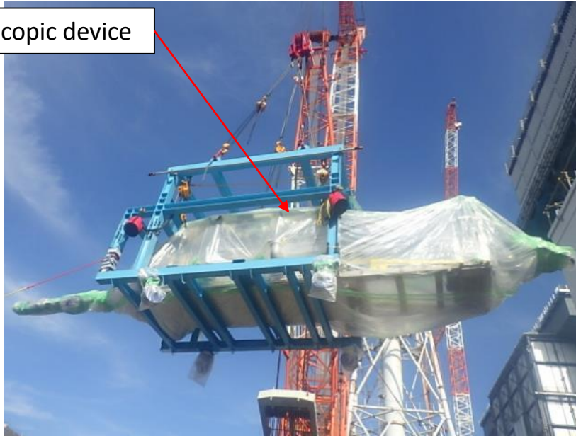
Removing the telescopic device from the reactor building (November 5)
