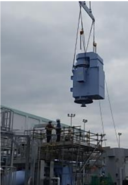
Lifting the electric motors
