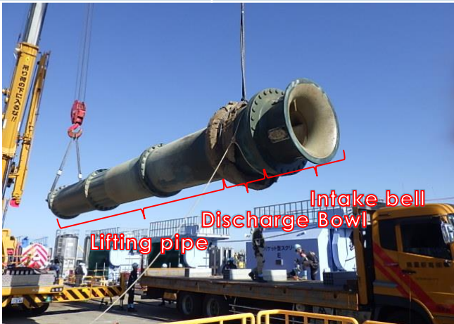
Lifting the pump
